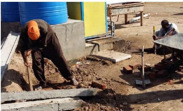
» Maintenance work at Shahpur Kanjran
